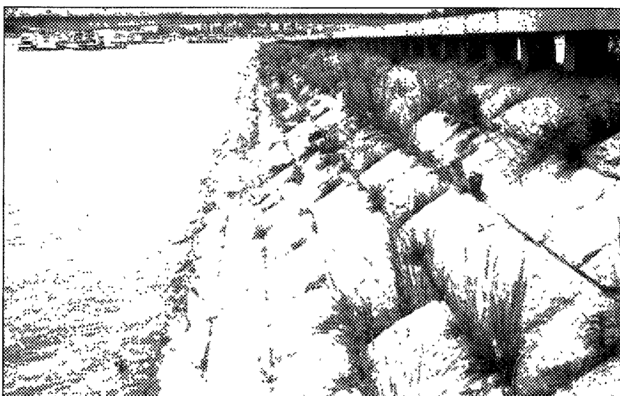
Figure 6. Streambank protection structures made of a wide range of stone sizes create more diverse habitat (a) than do those made of uniform concrete blocks (b). These structures can protect riparian vegetation from erosion. However, successional processes in the riparian are normally driven by flooding, erosion, and deposition. Photos from the Sacramento River in California.
